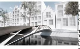
Royal HaskoningDHV, CEAD and DSM have announced that they have designed the first lightweight 3D printed FRP pedestrian bridge prototype using a composite material. It consists of a glass filled thermoplastic PET (<u>Arnite®</u>) and is combined with continuous glass fibres which are added in the 3D printing process. This unique combination offers high strength with extreme versatility and sustainability.
