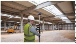
Racelogic is launching a brand-new indoor positioning system, called VIPS, which is an advanced system for measuring real-time 3D position to an accuracy of ±2cm in areas where GPS is not available, making it an ideal tool for construction applications both indoors and in urban areas. The system has been designed for any application that requires accurate measurement and recording of 3D positioning and enables GPS based technologies to operate in GPS denied environments.
